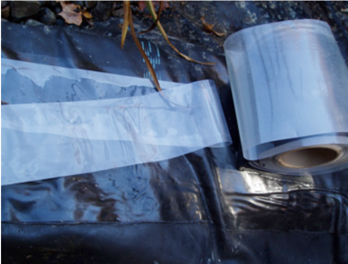
Remove the non-stick covering at the same time you are pressing the tape onto the liner. This eliminates the possibility of accidentally sticking the tape to itself, and minimizes airborne debris from attaching itself to the tape.
