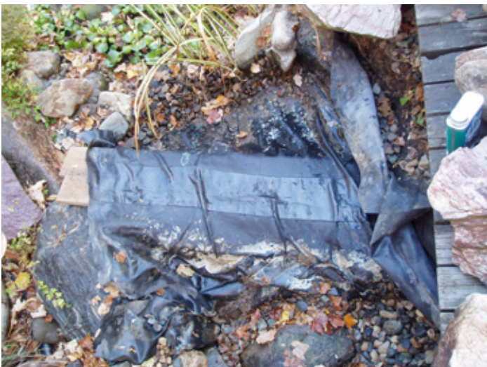
Completely clean & dry area, and place flat board underneath to provide a flat surface.
