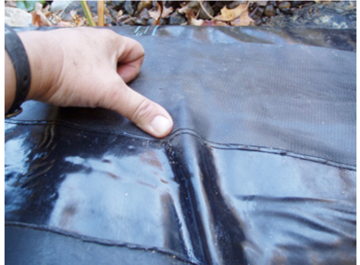
Pay particular attention to areas of the old liner that can't be flattened completely.
