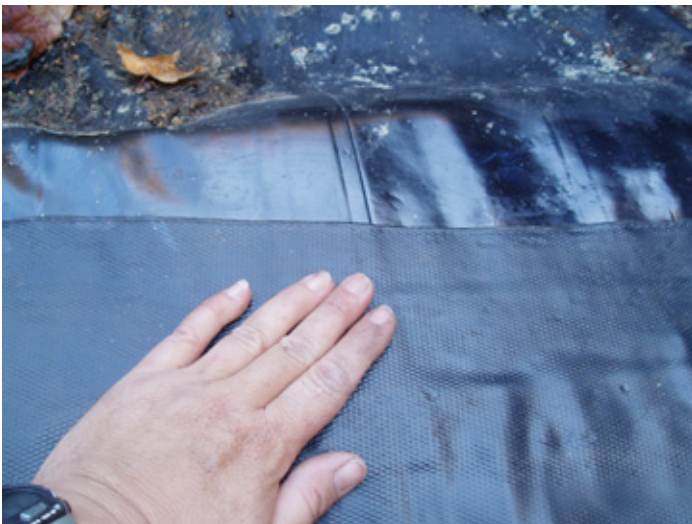
Press firmly to ensure good adherence, removing any bubbles or channels.
